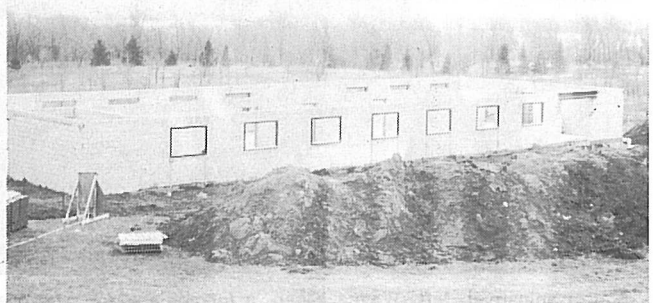
The completed first floor, awaiting Spancrete for the second floor.
