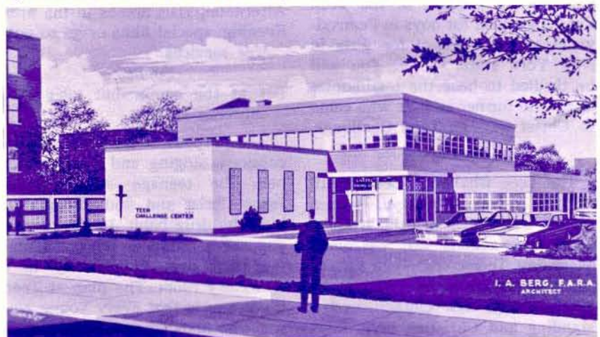
New building under construction
