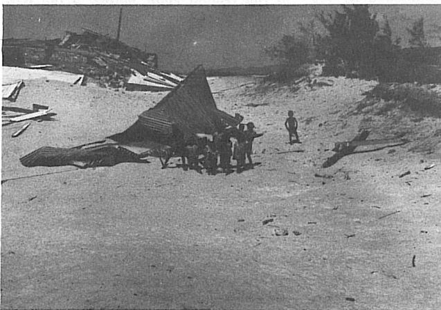
Antaninarenina Lutheran Church, completely destroyed.
