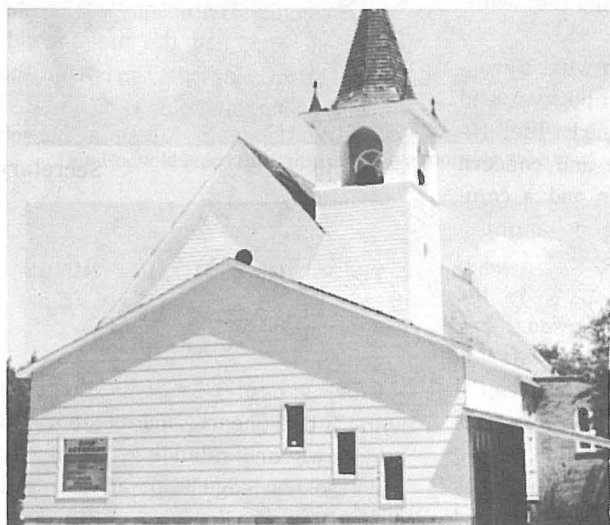
Zion Lutheran Church in Tioga, which was recently remodeled and the sanctuary and entry enlarged. The church also has a fine parish education unit, barely showing on the extreme right.
