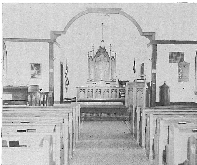
The interior of Bethany Lutheran
