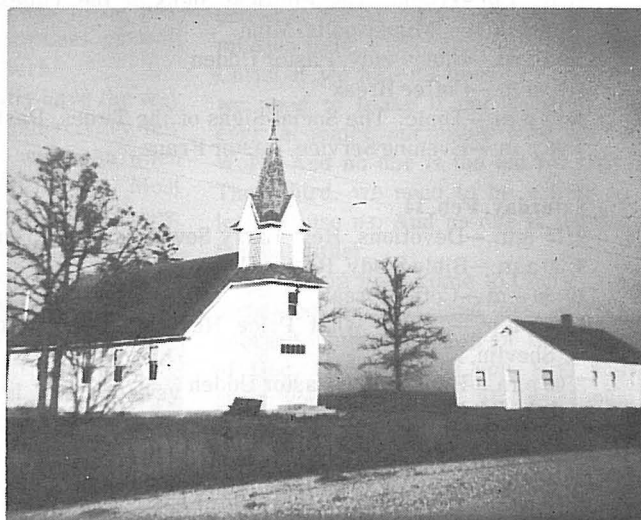
Zion Lutheran Church and Parish Hall
