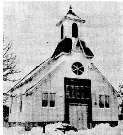
Westaker Church was placed on a foundation with a basement. Later this year an addition will be built on the far end of the church. The basement will provide room for a pastor's study.
