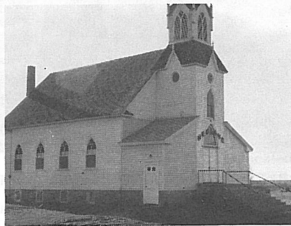
Hegland Church after two additions were made, on either side of the entrance. To the right are two washrooms with a furnace room in the basement. To the left is the ground-level entrance with stairways to the basement and main church floor. This also includes a cloakroom.
