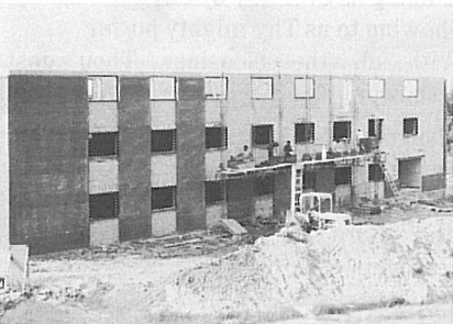
Exterior brick work being done.
