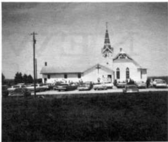
The remodeled Tabor Church. Note the parish hall on the left and the ground-level entry.
