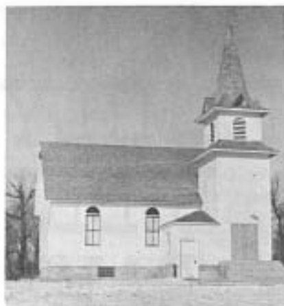
Aspelund Lutheran Church, Langdon, N. Dak.
