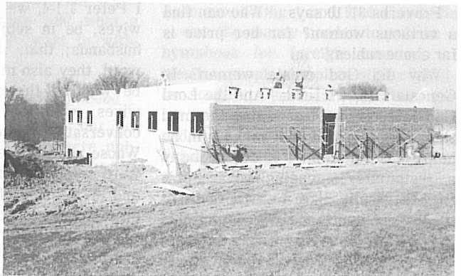
Work on the second floor of the new dorm.
