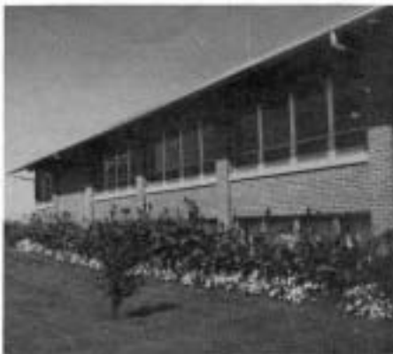
The Girls' Dormitory in the Headquarters Building (Basement)
