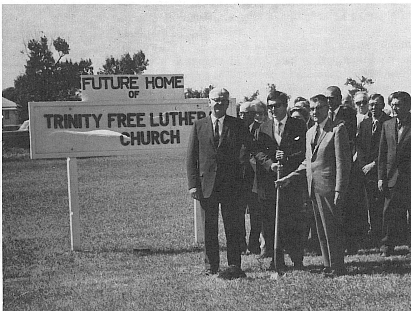
Groundbreaking for Trinity Lutheran Church
