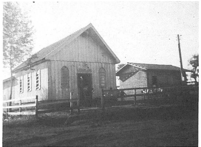
At the right is the Evangelical Primary School. To the left is the Lar Parana church showing the new addition at the rear.
