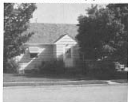
This is the parsonage occupied by the Reuben Wees. Acquired this year, the house is at 310 N. Main St., just north of Zion church in Tioga.
