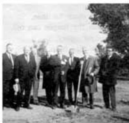
Ground-breaking at Culbertson, Montana. From left to right: Erling Brekke, Henning Dahlberg, Orville Qualley, Kinley Salstad, Clifford Berglee, Otto Hansen, Pastor Jore and Paul Jacobs.
