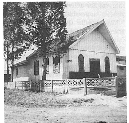
Lar Parana Church, with the new cement fence.
