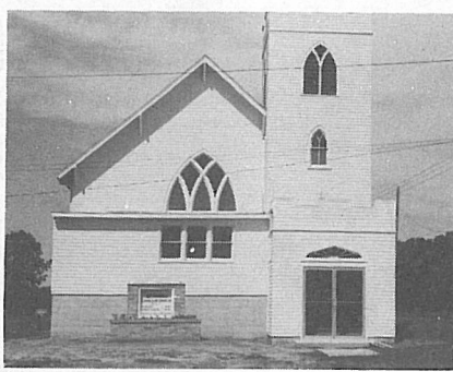
The completed building from the outside.
